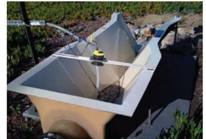
determine its volume, content and risk to the local environment. Here, an EchoPod ultrasonic level sensor is installed over a V-Notch weir on the side of the highway. The continuous level sensor measures the volume of stormwater passing through the weir, and provides a 4-20 mA signal to the wireless telemetry system for remote data collection.
